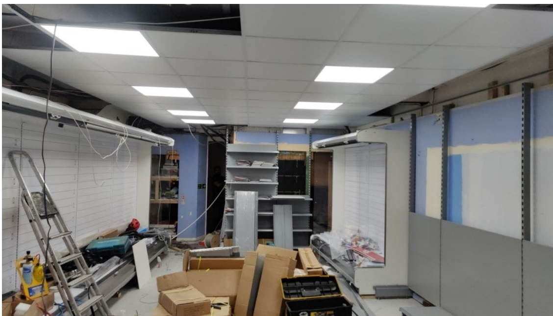
Picture showing refurbishment (above)
